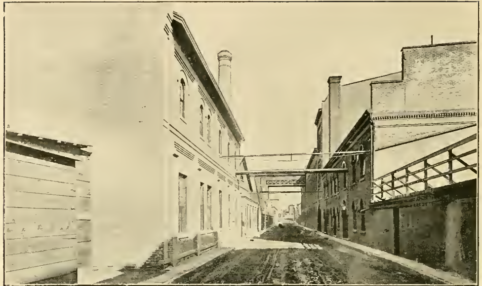
VIEW OF THE PLANT OF THE NEWARK GAS LIGHT CO., ON JERSEY STREET.
